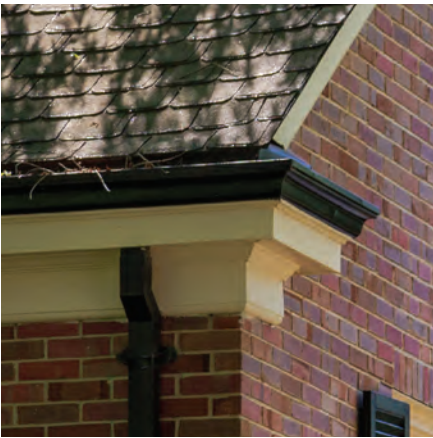
ROOF MATERIALS & EAVES
