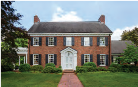
Symmetrical and balanced façades
