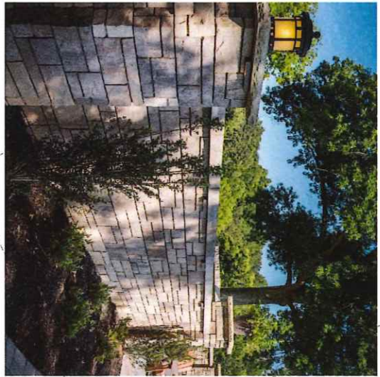
FRONT SIDEWALK WALL DETAIL (INDEPENDENT WALL SYSTEM) MAXIMUM 3-FT HEIGHT OF WALL WITH 16" TALLER COLUMN AT EACH END
