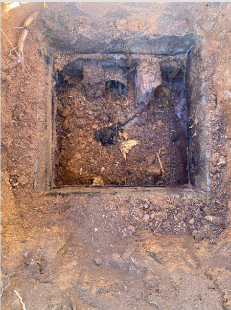
Outlet side of tank.
