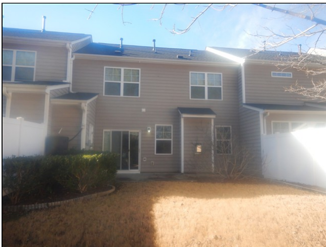
2.0 Item 6(Picture) Rear of house
