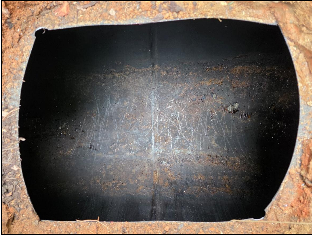
Photo 3. View of the UST interior after the removal of UST contents and pressure wash cleaning of the tank interior.
