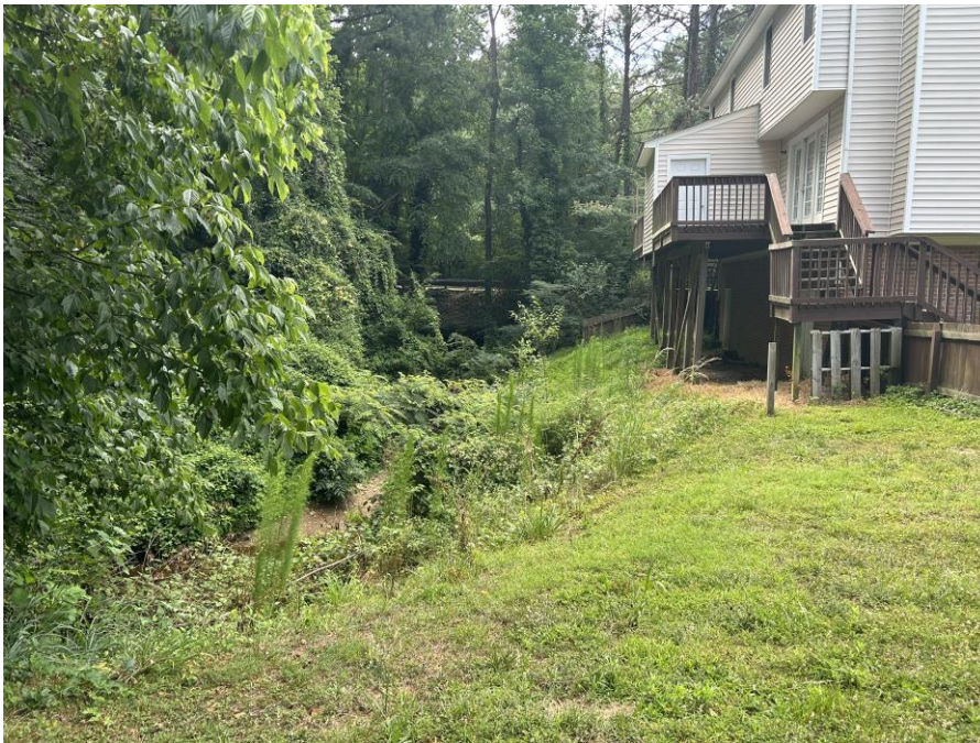
Photo 2: Fill slope behind 500 and 502 Brent Rd
