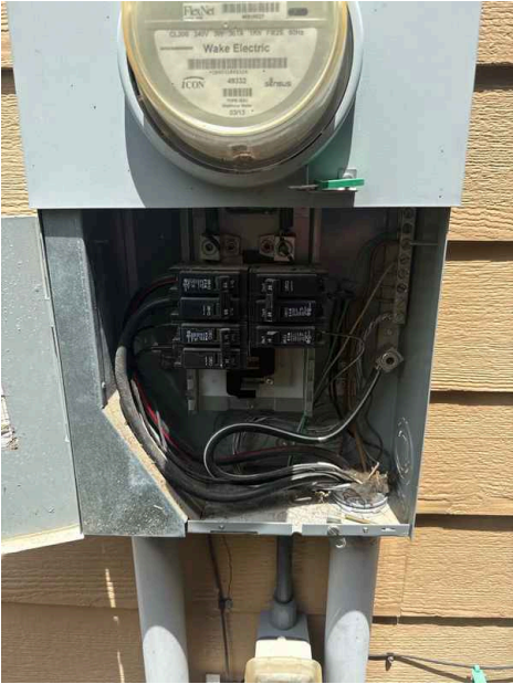
Main Panel: Electrical Service Ampacity 200 AMP
