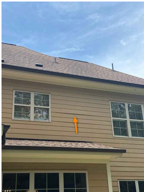
Laundry Rear Left 2nd Floor
