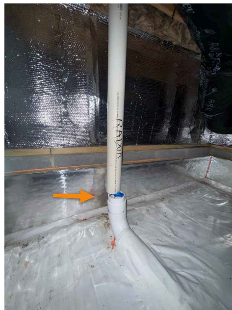
Rear Left Crawlspace
