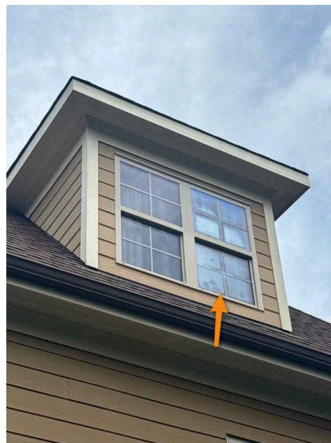
Attic, Right Exterior
