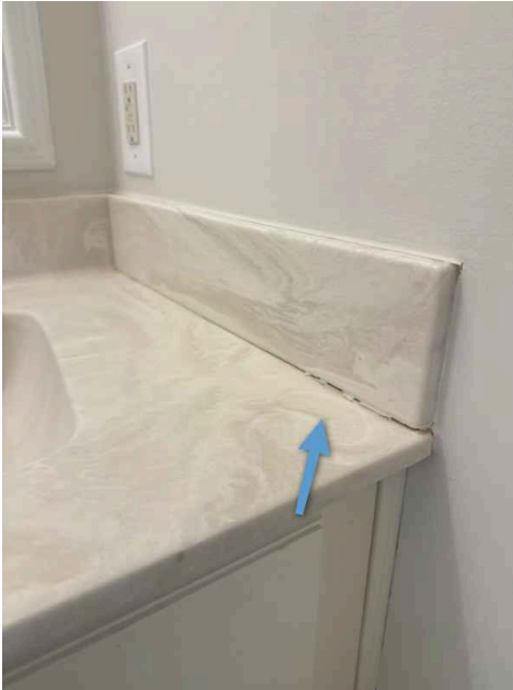
2nd Floor Shared Bathroom
