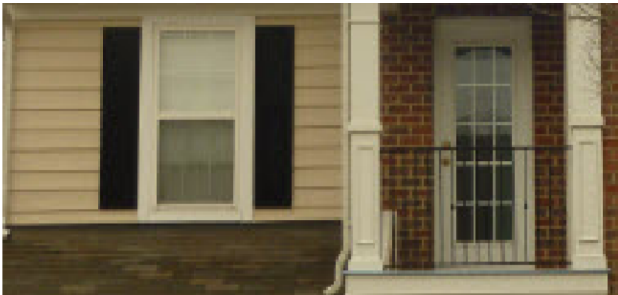
Example of Shutters
