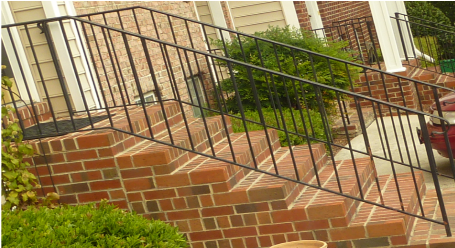
Example of Railings and stairs
