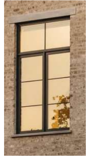
STONE CASING AND LINTELS
