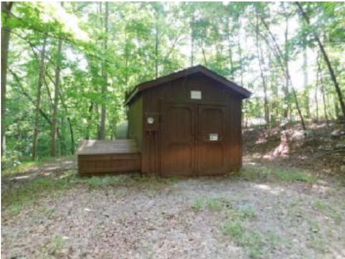
Community well house
