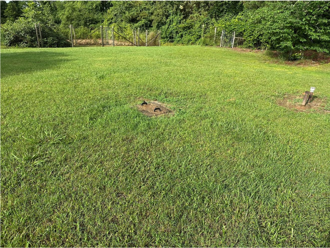
Septic Tank Location
