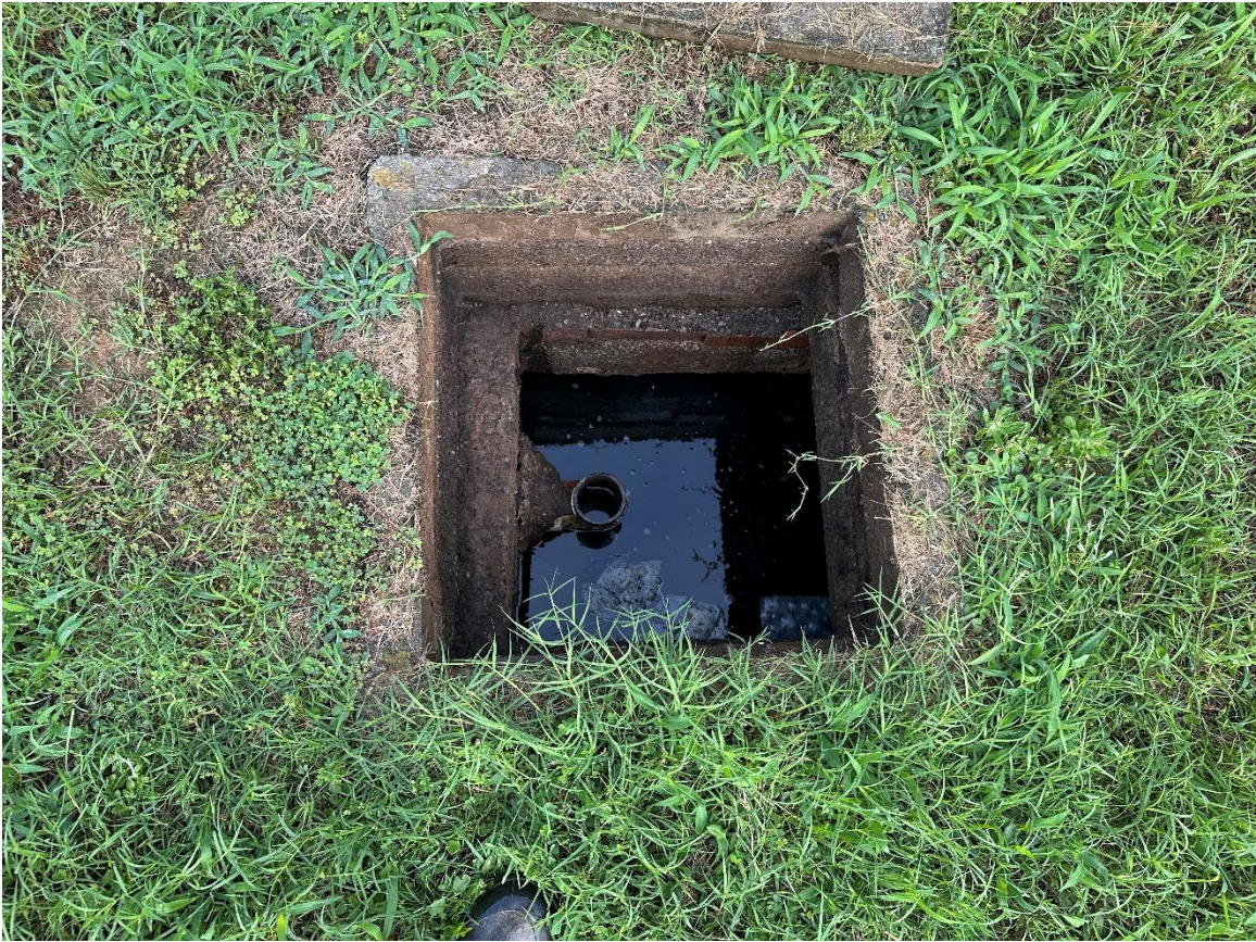
Outlet Access Point of the Septic Tank
