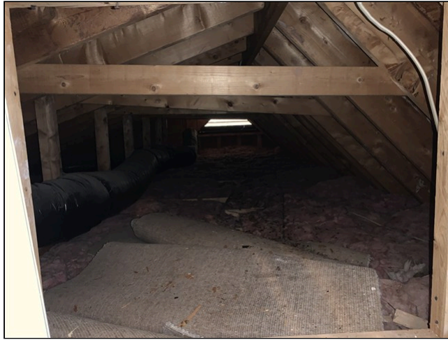
4.6 Item 5(Picture) Attic area to right of third floor not entered due to lack of clearance and lack of flooring
