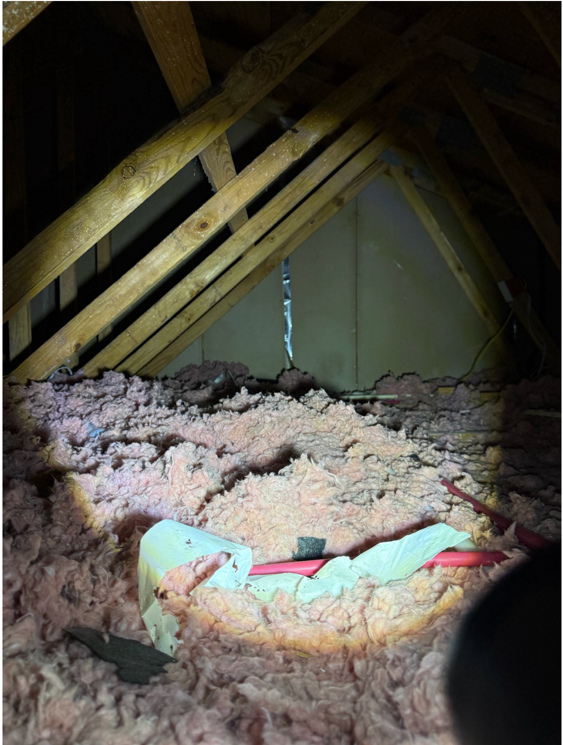
PICTURE 2 – ROOF TRUSSES WITH CONSISTENT PROFILE ACROSS LOCATION WITHOUT WALL AND WHERE WALL WAS REMOVED
