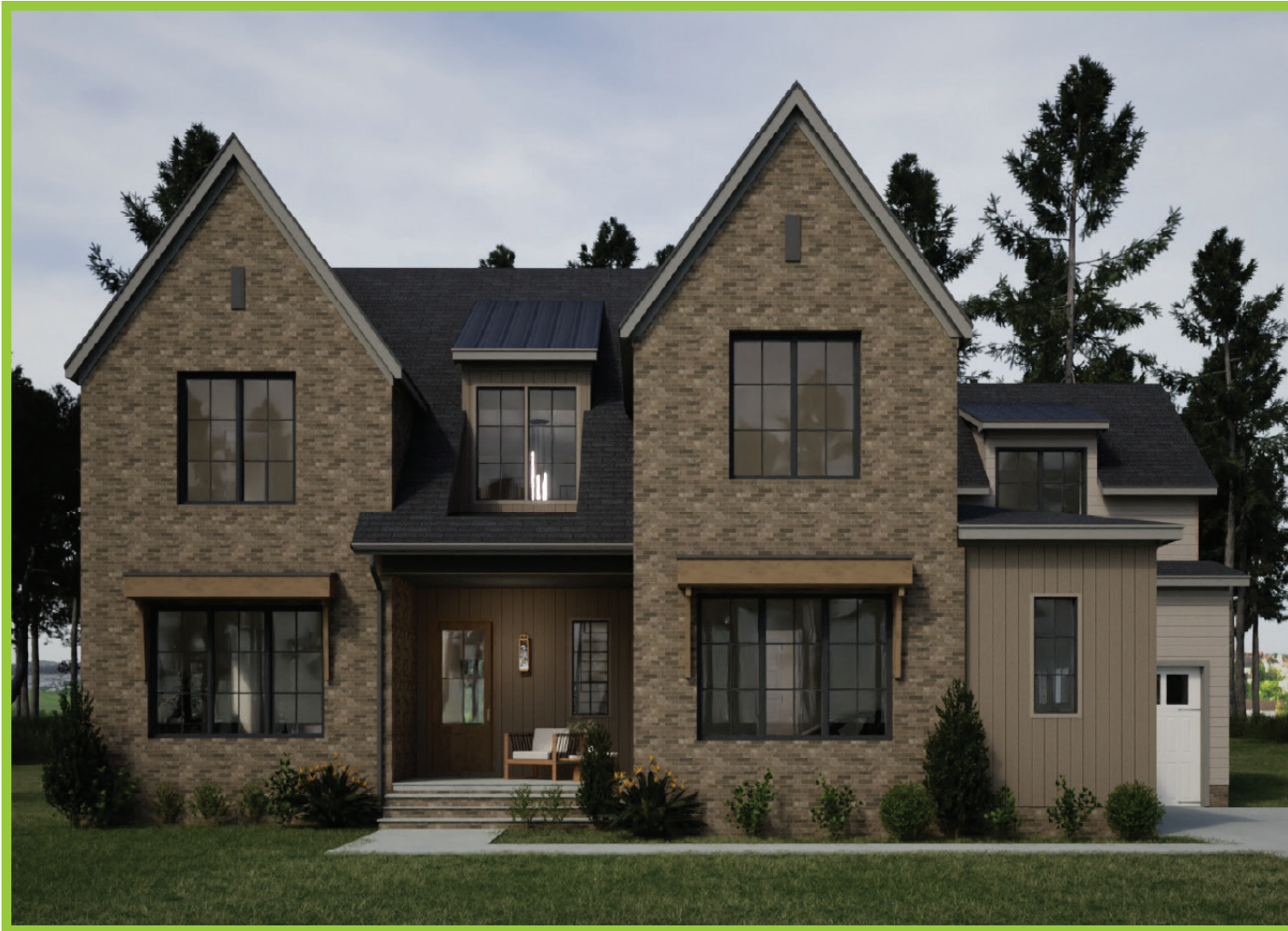
HOMESITE 28 BY THAYER HOMES
