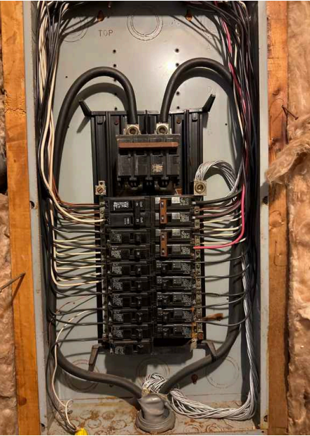
Main Panel: Electrical Service Ampacity 200 AMP
