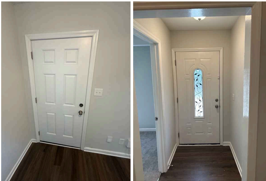
Photo - Exterior Door - Inside
