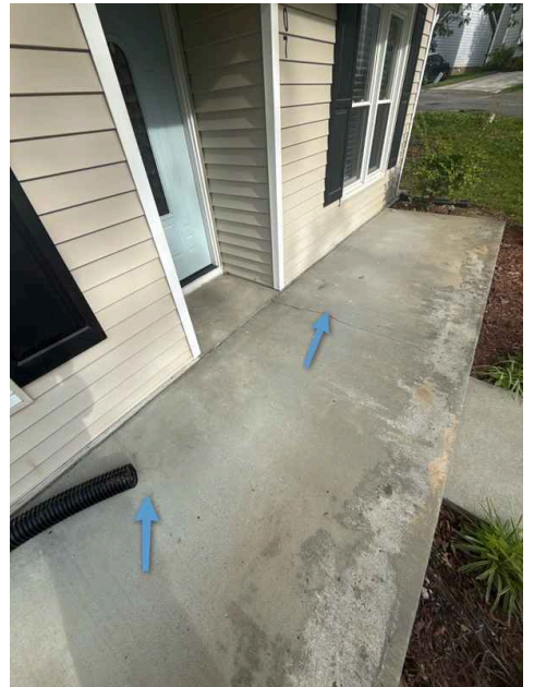
Living Room Front Exterior
