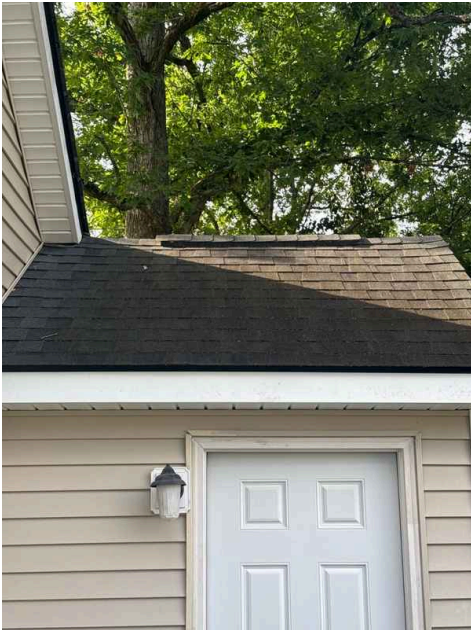
Rear Roof (moss)
