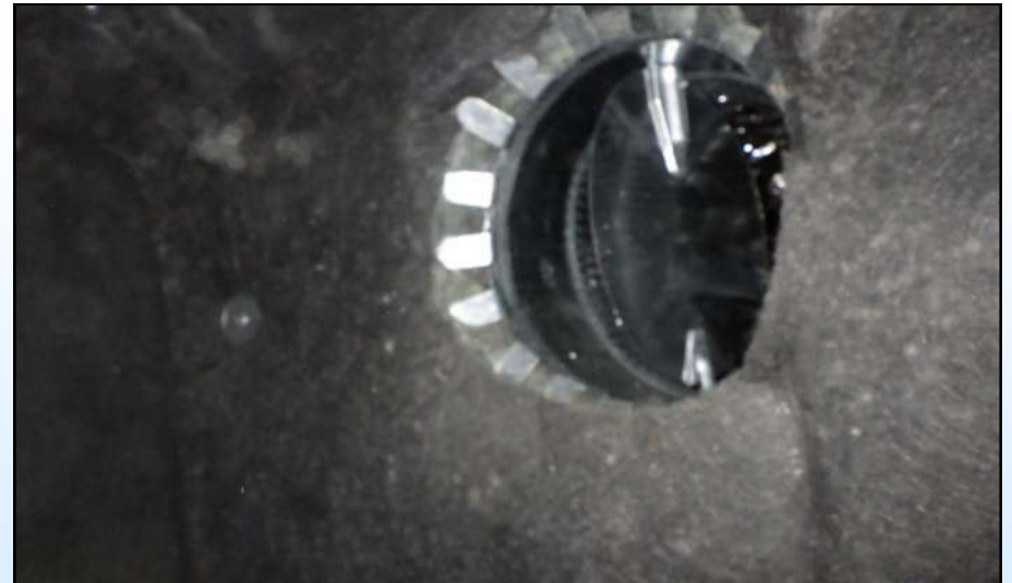
The attached distribution box was checked—looks clean.
