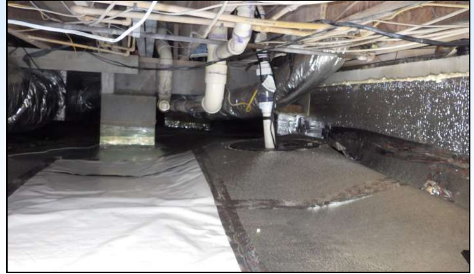
Crawlspace looks good and is performing well!
