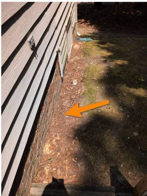
Back of home, negative grading - during a heavy rainfall, check the effectiveness of the gutter system
