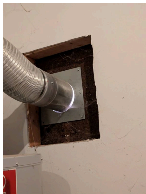
Vent should be sealed with fireproof sealant
