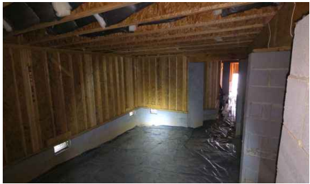
Basements & Crawlspaces: Method of Inspection Walked/Crawled, Flashlight, Probe
