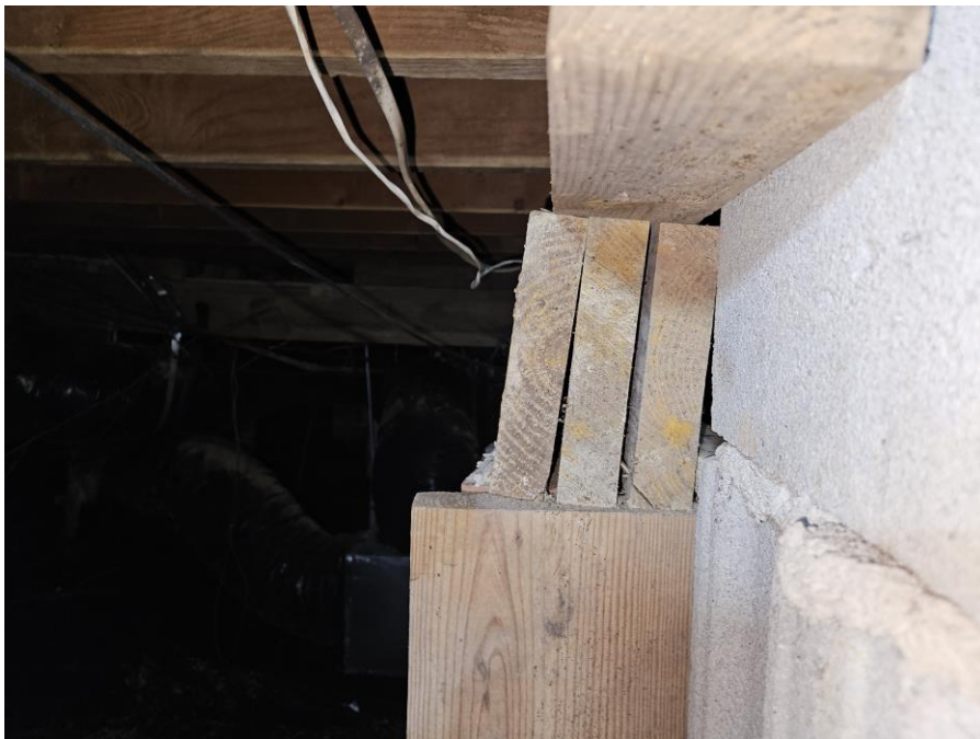
Picture 8 – Rotated and separated plies
