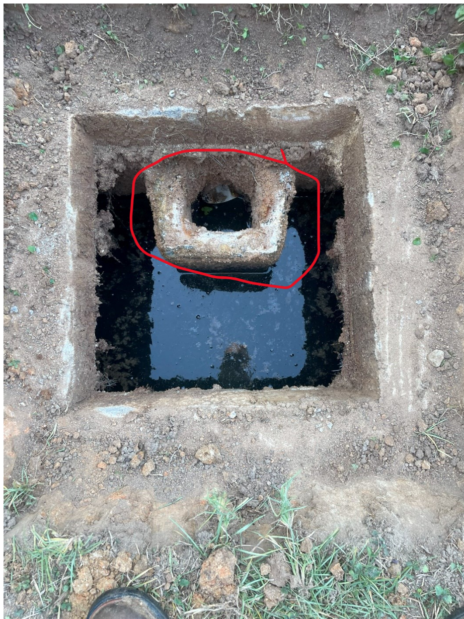
This is the outlet end of the septic tank with the outlet tee. The outlet tee is in good condition.
