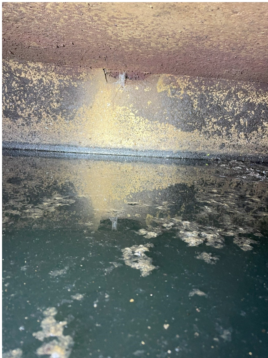
This is the inlet end of the septic tank. The tank does not need to be pumped.
