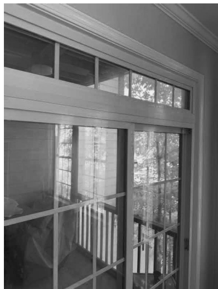
Rear sliding door and transom
