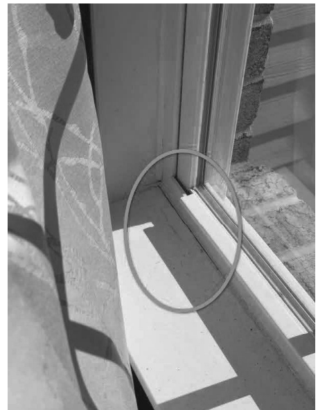
3rd floor front bedroom windows
