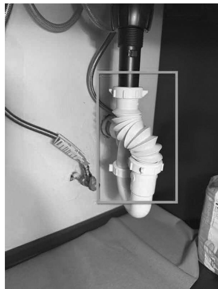
3rd floor hall bath sink drain
