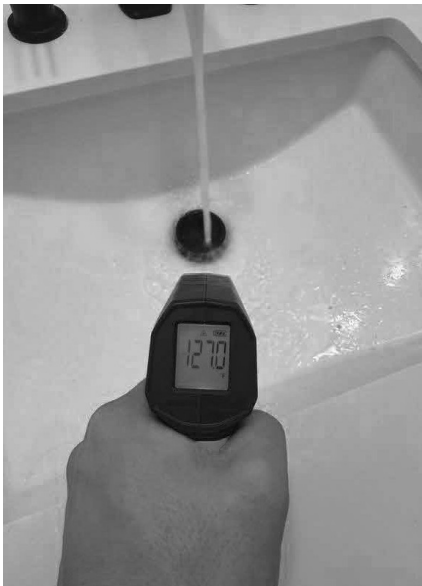
Water heater supply temp
