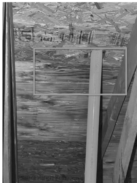
Rear roof, at plumbing vent penetration. Tested dry at time of inspection
