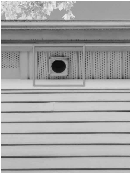
Rear soffit area
