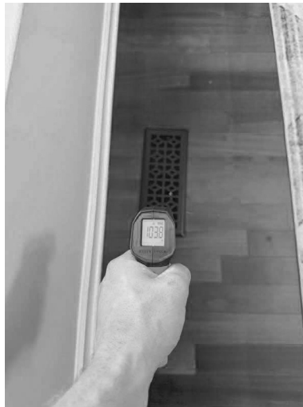
2nd floor heating supply temp
