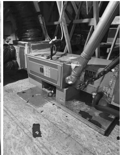
Located in attic area
