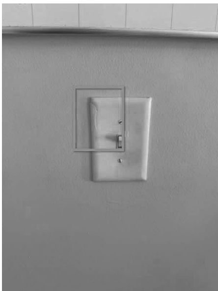
3rd floor front bedroom
