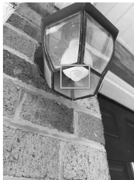
Multiple exterior fixtures
