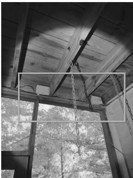
Rear deck areas
