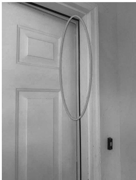
Garage entrance door. Rubbing frame
