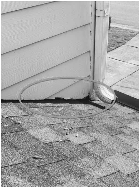
Front porch roof
