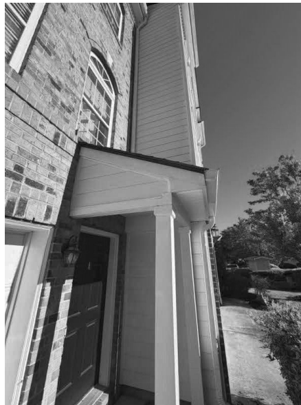
Fiber cement siding
