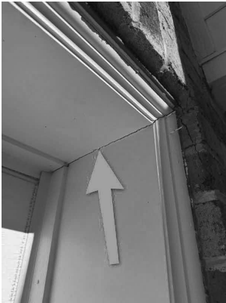
Garage door surround trim
