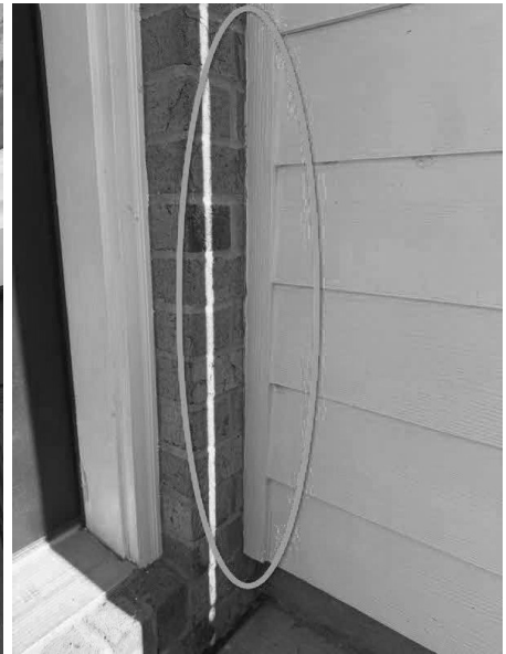
Front porch area
