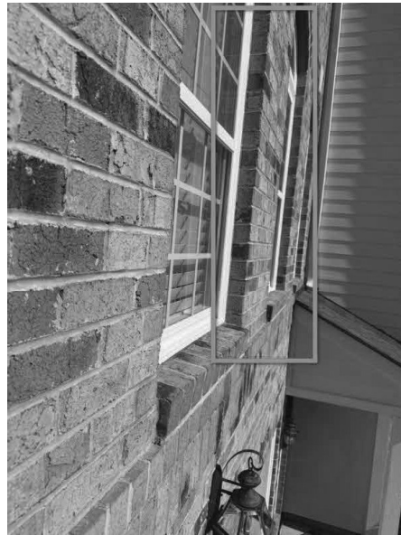
Multiple window perimeters at front exterior
