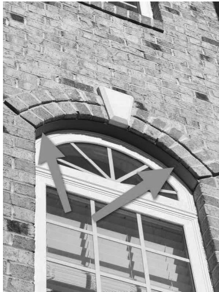
Front exterior window lintels
