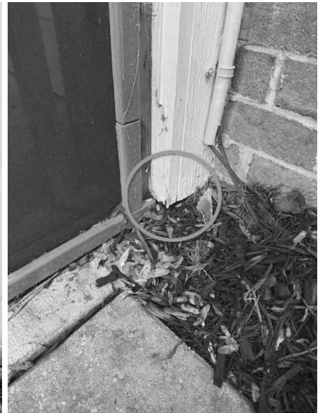
Rear patio patio corner trim
