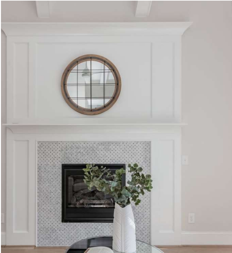
Traditional Fireplace Insert Raised 12" off floor with Mantle and Tile Surround
