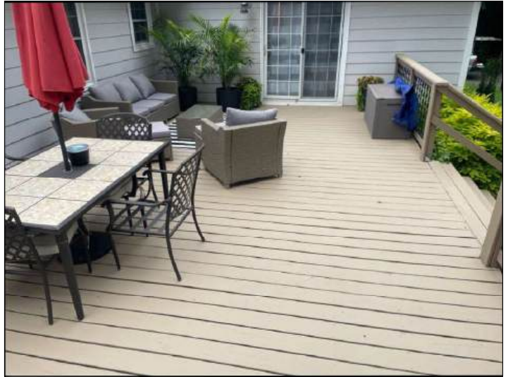
The deck walking surface
