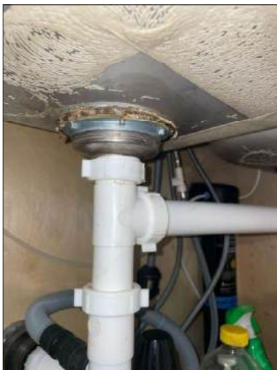
There are leaks around the kitchen sink left basin basket fitting.
