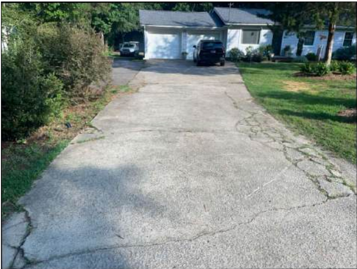
The concrete driveway
