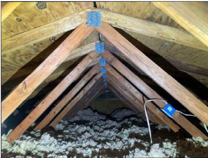
A general review of the roof structure
