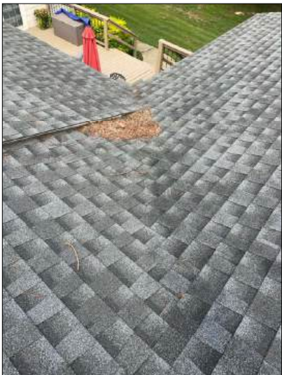
The roof valleys on this home are configured as woven. Roof valleys should be kept clear of organic debris.
