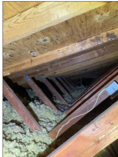
A general view of the roof structure
