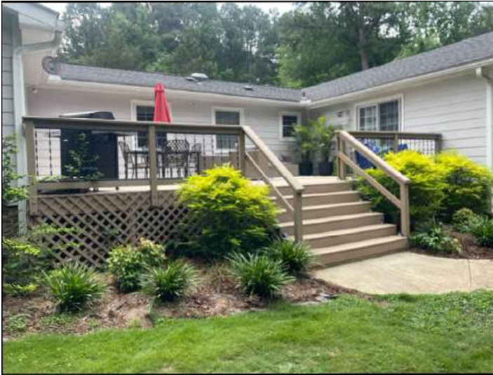
The deck structure
