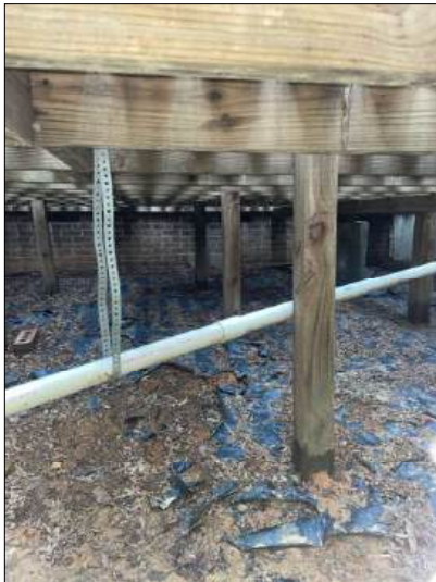
There are several supplemental support posts below the deck, which are commonly referred to as a stiff knee.
