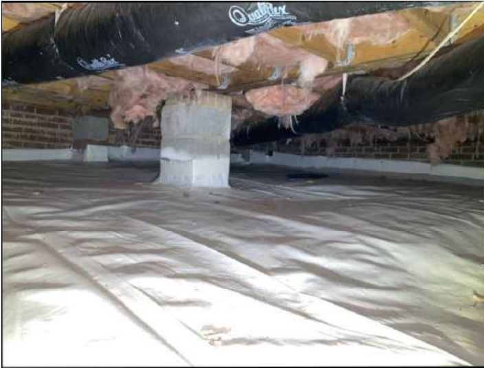
A general view of the right side crawlspace, below the primary bedroom area
