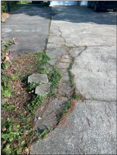
Broken concrete
