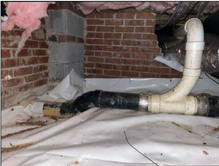
The main waste line exits the home envelope as ABS, at the rear side right of the left crawlspace.
