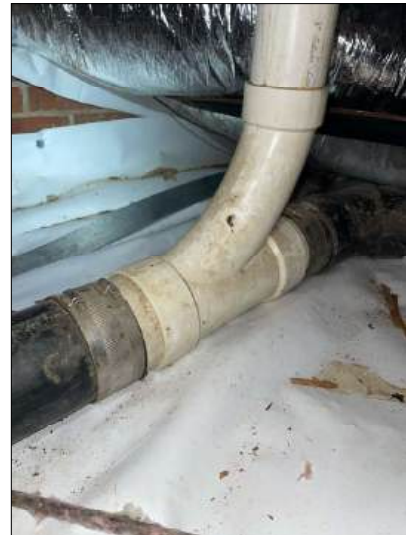
This photo shows the proper mating of PVC to ABS pipe, using coupler fittings.
