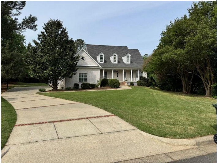
Photo 1: Front view of the home
