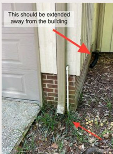
Right front corner
