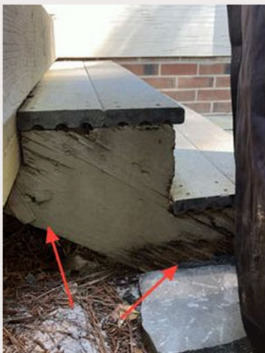
Rear deck steps
