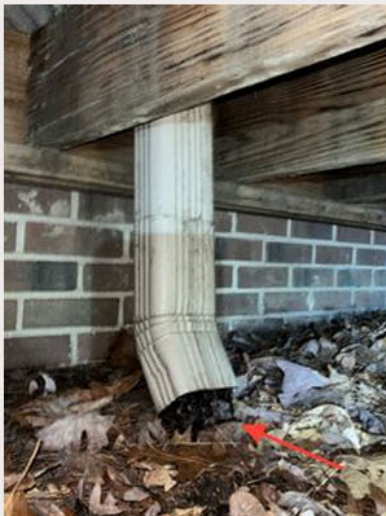
Under deck at rear side of unit
