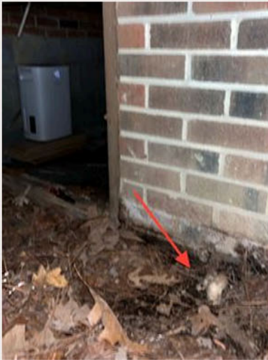
Condensate drain for air conditioning system
