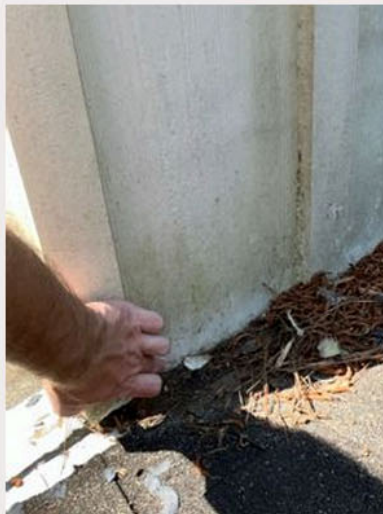
Damaged siding/trim
