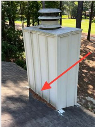
Add a "cricket" when reroofing
