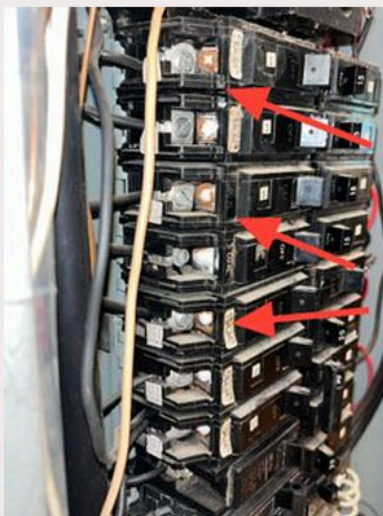
Some corrosion was noted on the older circuit breakers
