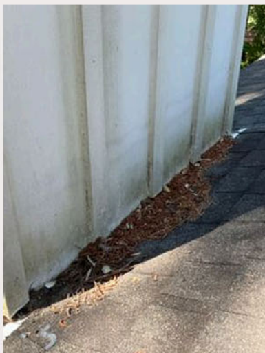
Front side of chimney
