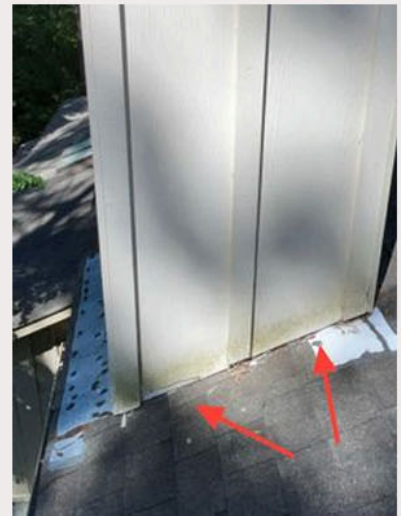
Left side of chimney chase
