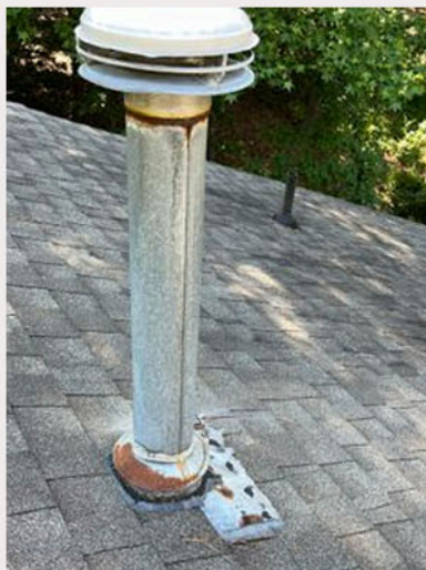
This is a very old furnace flue that should be replaced
