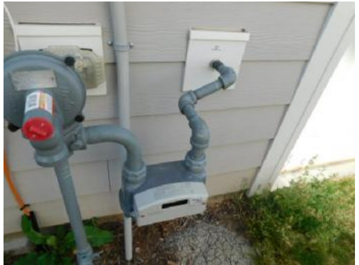
HS-9 (Pg 5): No visible bond at the exterior
