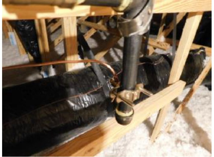
HS-9 (Pg 5): Bond at the manifold in the attic
