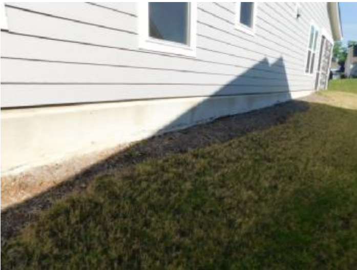
Concrete slab foundation
