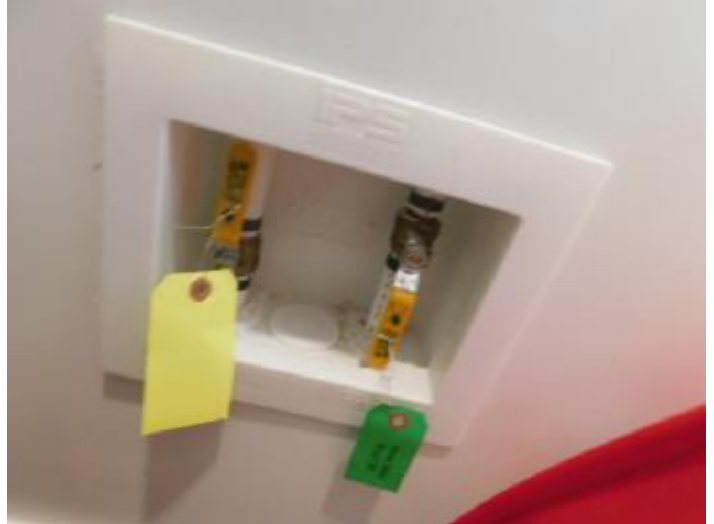
Main water shut off
