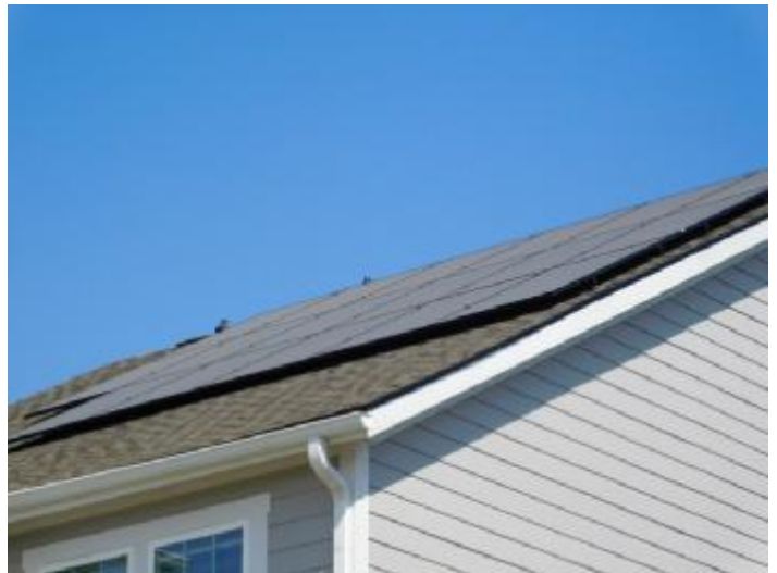
Solar panel system
