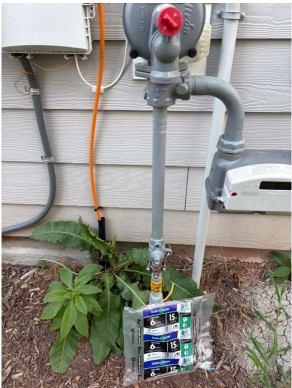
Bonding clamp detail
