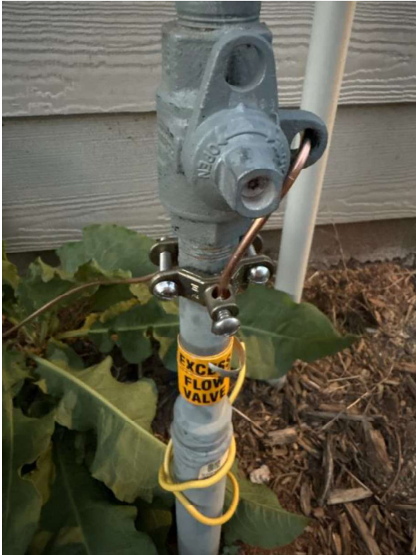
Bonding clamp detail
