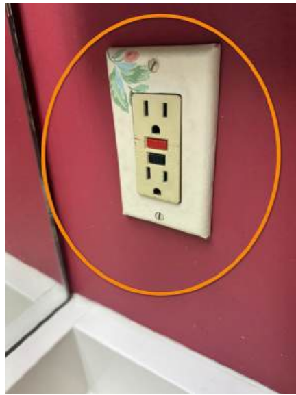
The GFCI receptacle in the did not work/trip off when tested at the time of inspection (main level primary bathroom)
