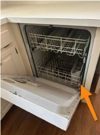
The dishwasher is not secured properly and has movement
