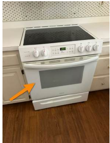
The range did not appear to have an anti-tip device installed
