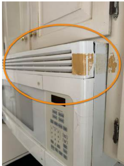
Microwave exhaust vent cover is damaged/detaching
