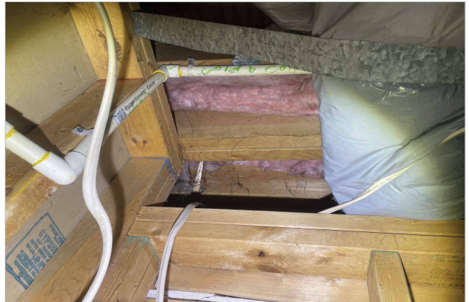
Basement insulation, floor joists and water pipes
