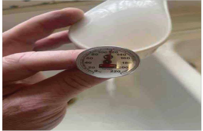
Hot water temperature
