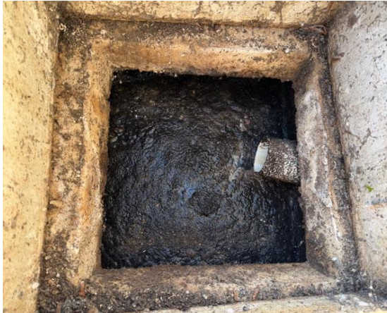
Inlet chamber shown open for inspection
