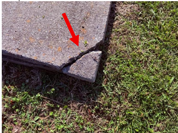
Pump chamber riser lid shown broken
