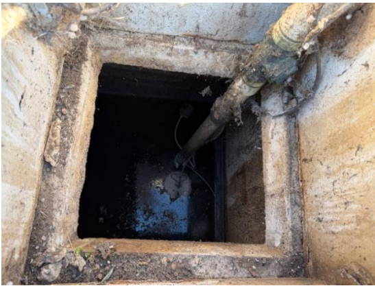
Pump chamber electrical junction box shown inside of pump chamber. Conduit not sealed
