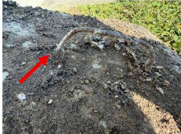
Inlet chamber lid handle shown broken
