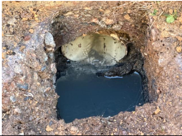
Pump chamber riser lid shown broken
