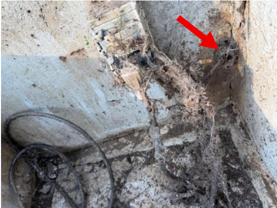
Pump chamber electrical junction box shown inside of pump chamber. Conduit not sealed
