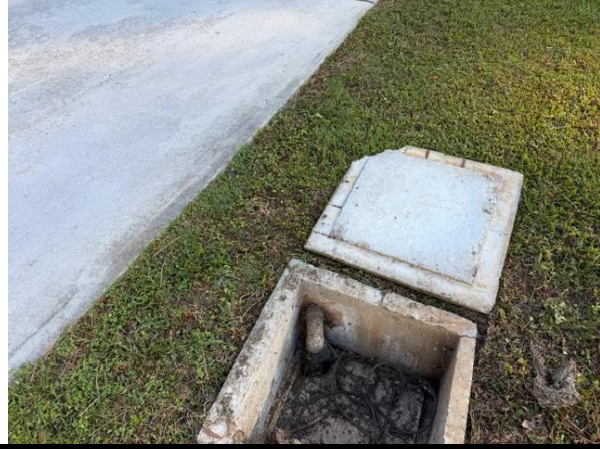
Pump float noted as not being properly attached to float tree
