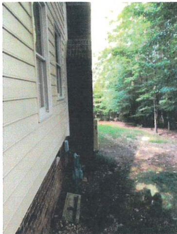
Side view of lower part of chimney
