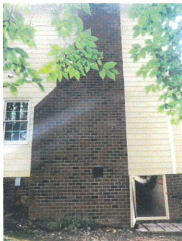
Front view of chimney
