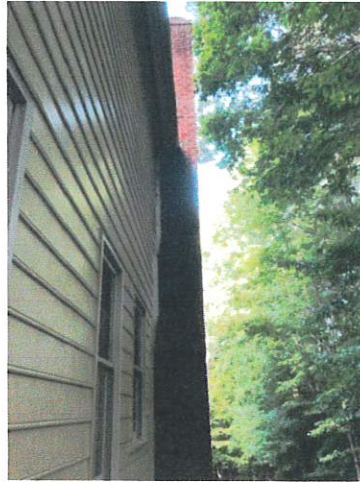
Side view of chimney
