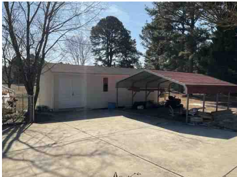
STORAGE1 AND CARPORT
