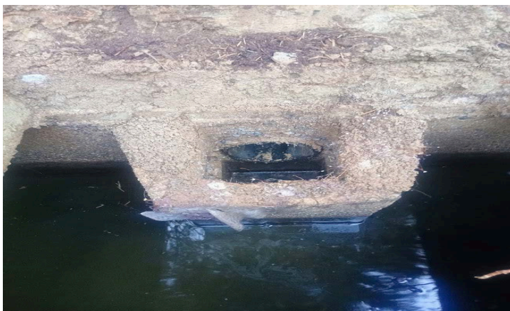
Below normal effluent level shown
