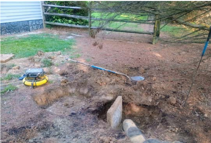
Minor sludge are roots in the leach field lines
