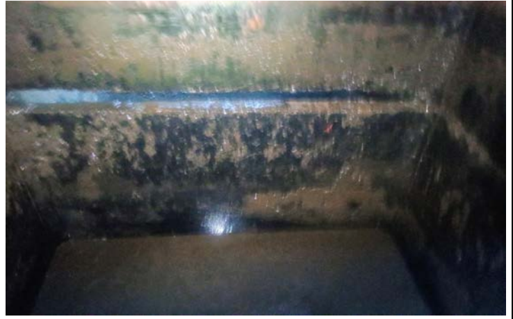
No visible cracks inside of the septic tank
