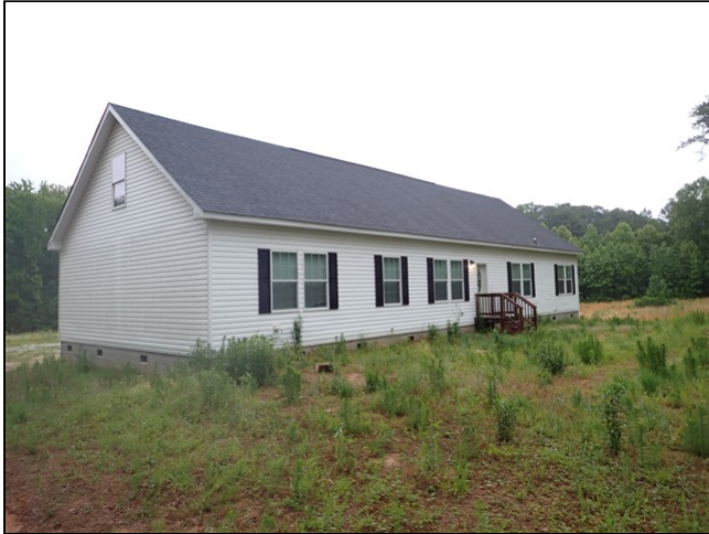
2.0 Item 3(Picture) Left front corner of house
