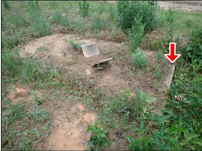
4.0 Item 2(Picture) Exposed top of septic tank
