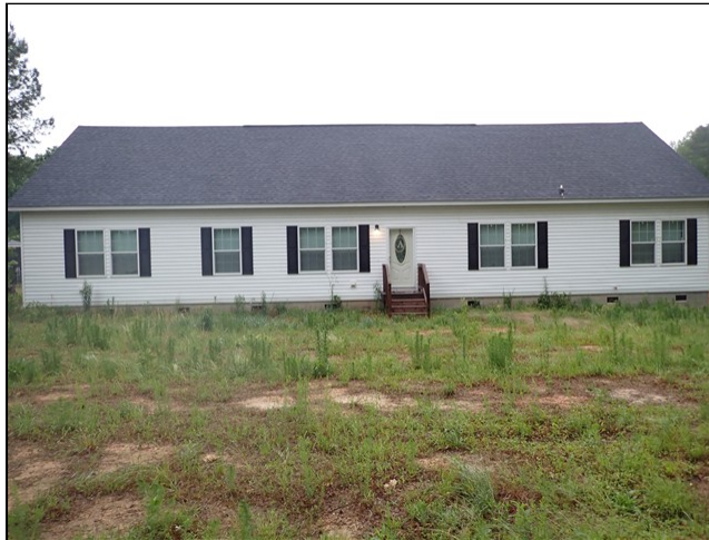
Front of 235 Joe Ayscue Road
