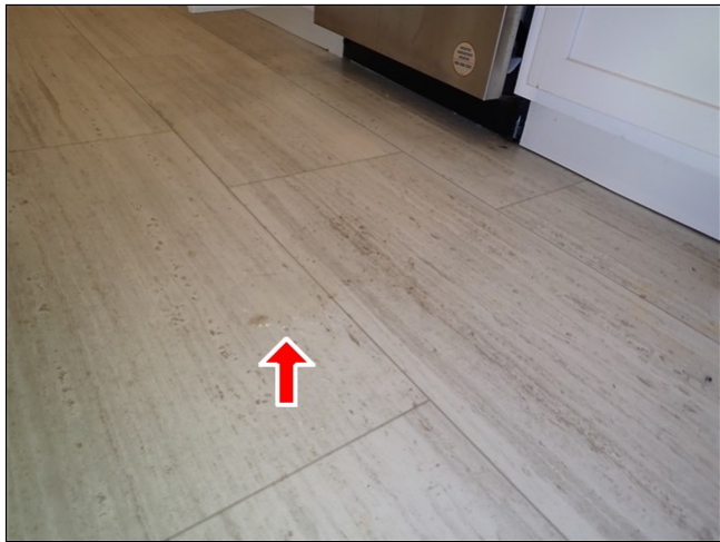
10.0 Item 1(Picture) Puddled water
