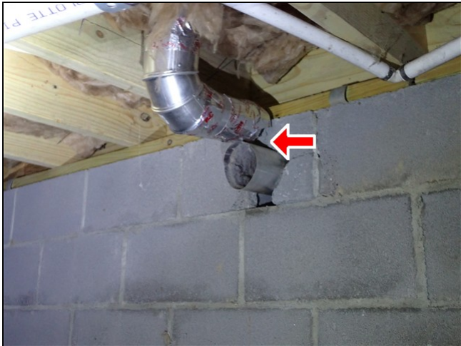
9.4 Item 1(Picture) Separaed dryer exhaust tube
