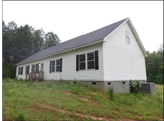
2.0 Item 4(Picture) Right front corner of house
