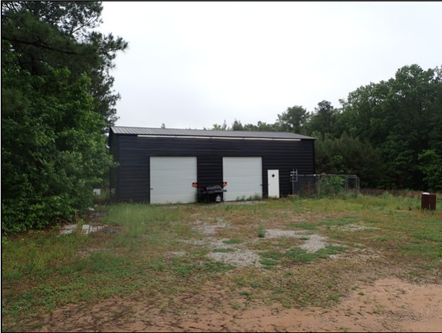
2.7 Item 1(Picture) Detached garage
