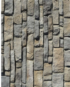
Front Foundation Stone
