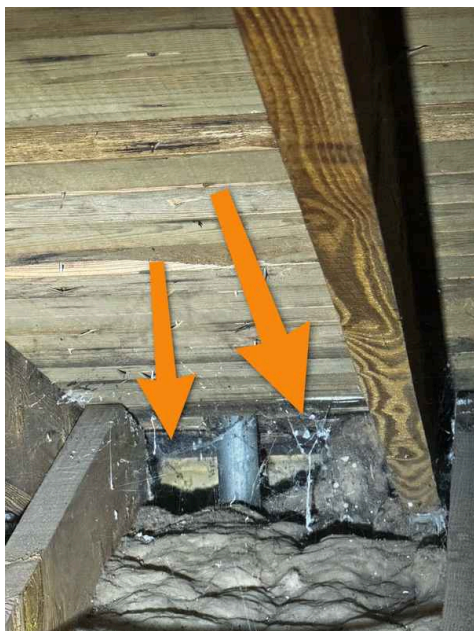
Additional photo of this finding showing decay from inside the attic.
