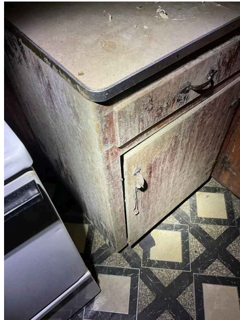
Additional photo of this finding.
