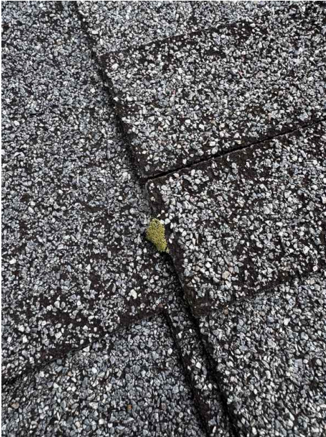
All areas of the roof should be assessed for the same finding.
