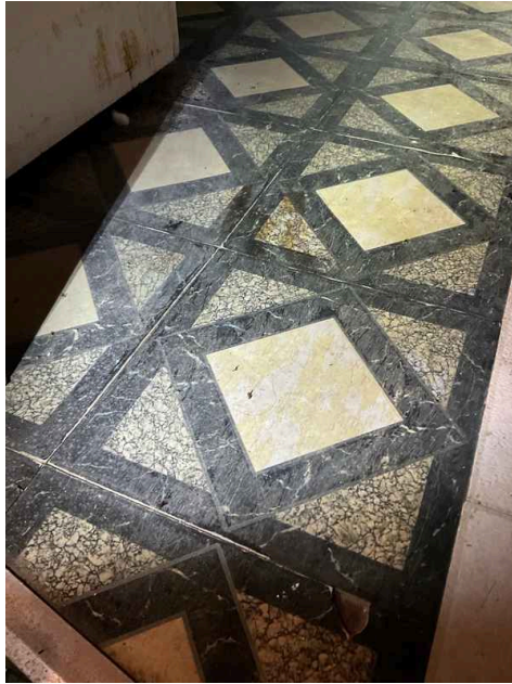
Based on the dimensions of the tile and age, these are likely asbestos as well.
