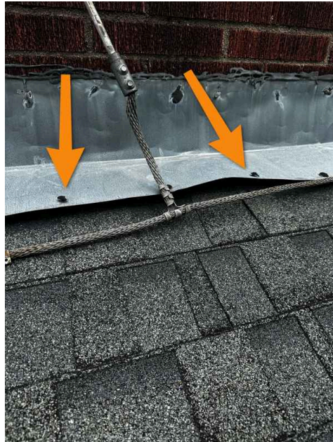
Additional photo of this finding showing more loose flashing.
