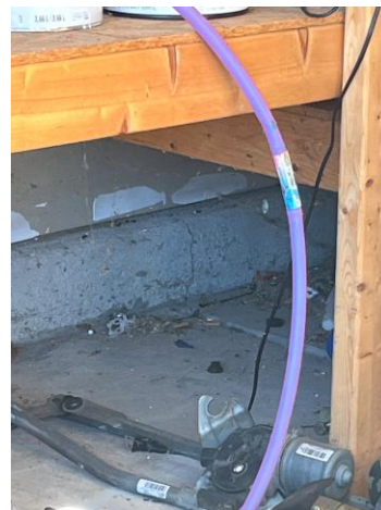
Picture 4 – Foundation crack
