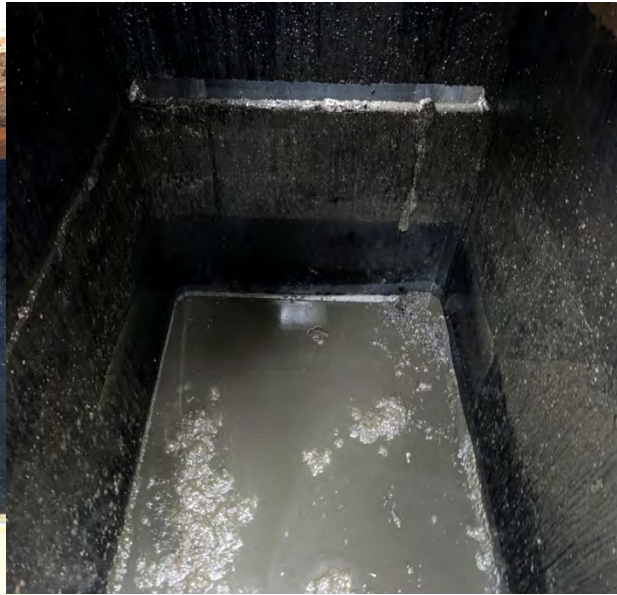
Inlet side after pumping
