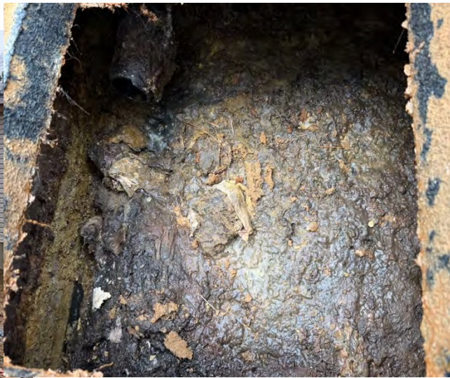
Inlet side of septic tank before pumping
