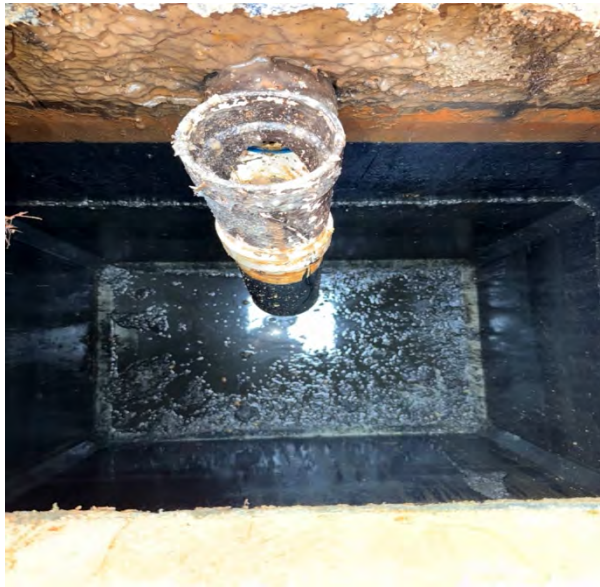
Outlet side of septic tank before pumping
