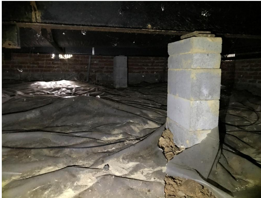
View of interior pier and strap anchorage.
