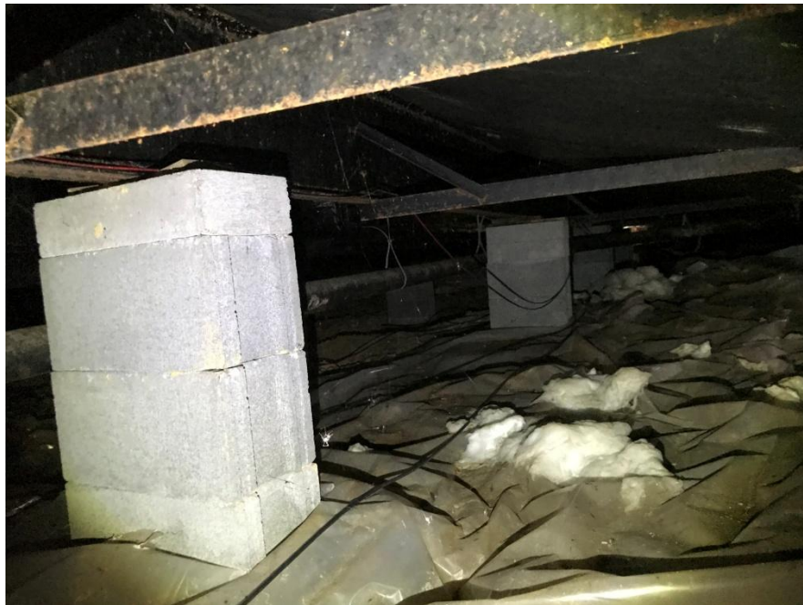
Crawl space view of interior piers
