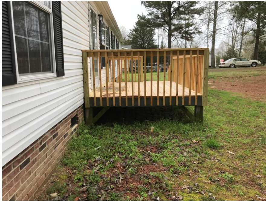
View of front free standing detached deck.
