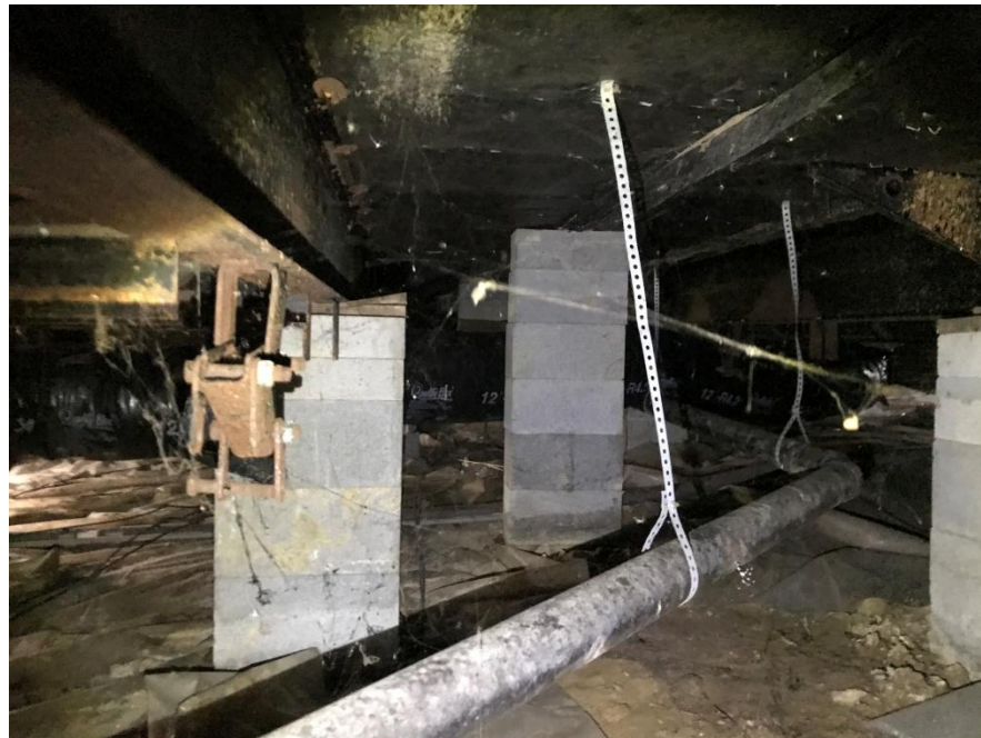
View of interior piers and center joint marriage piers.
