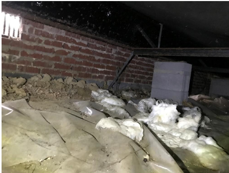
Crawl space view of brick masonry curtain wall, perimeter piers, and anchor straps.
