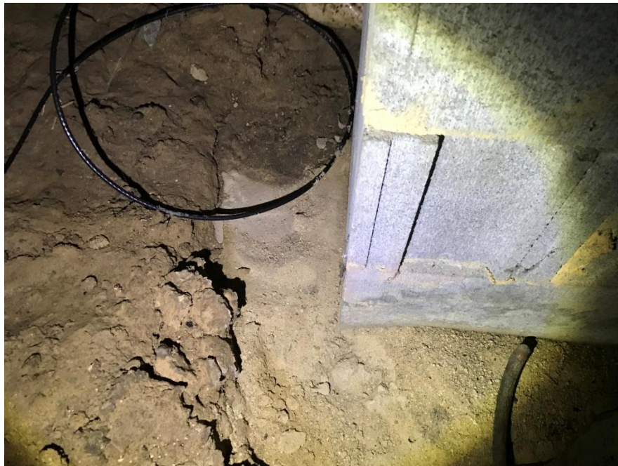
View of interior pier on footing.
