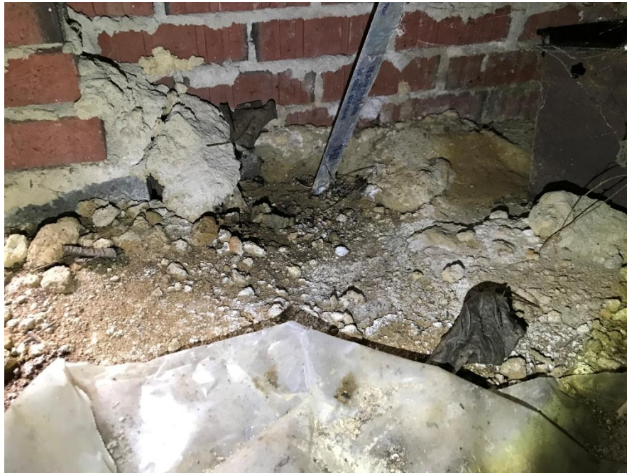
Crawl space view of strap anchorage into concrete
