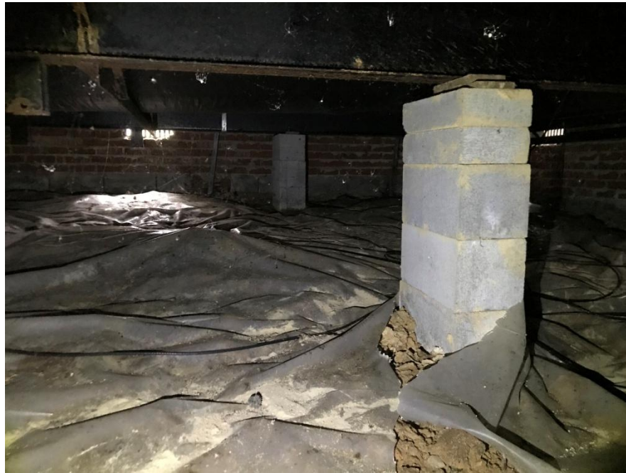
Crawl space view of interior piers
