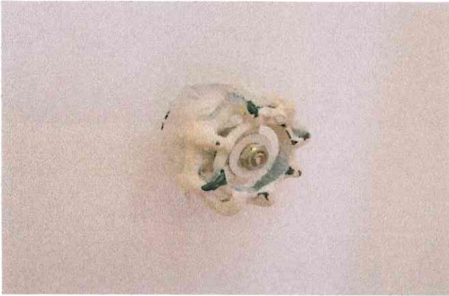
Main water shutoff valve shown where installed in the closet under the stairs
