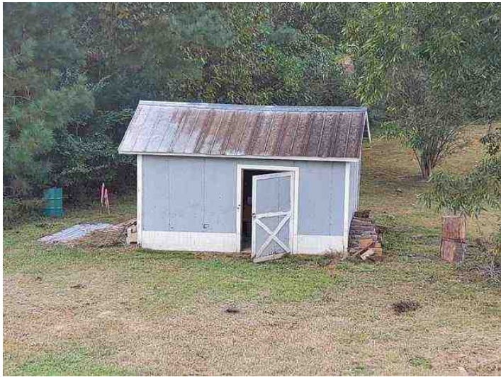
Detached Storage Shed
