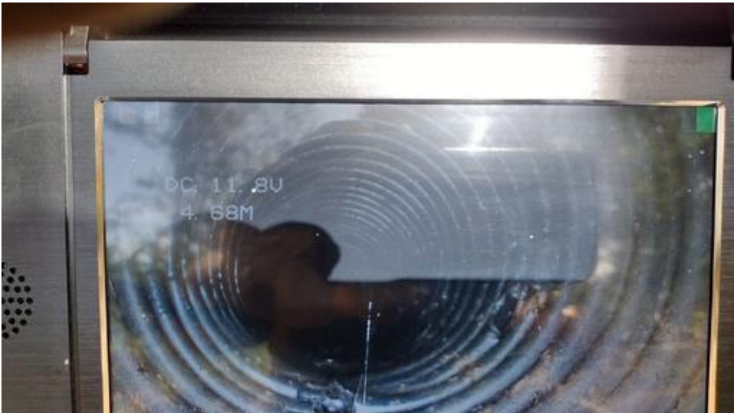
DRAIN LINES through CAMERA
