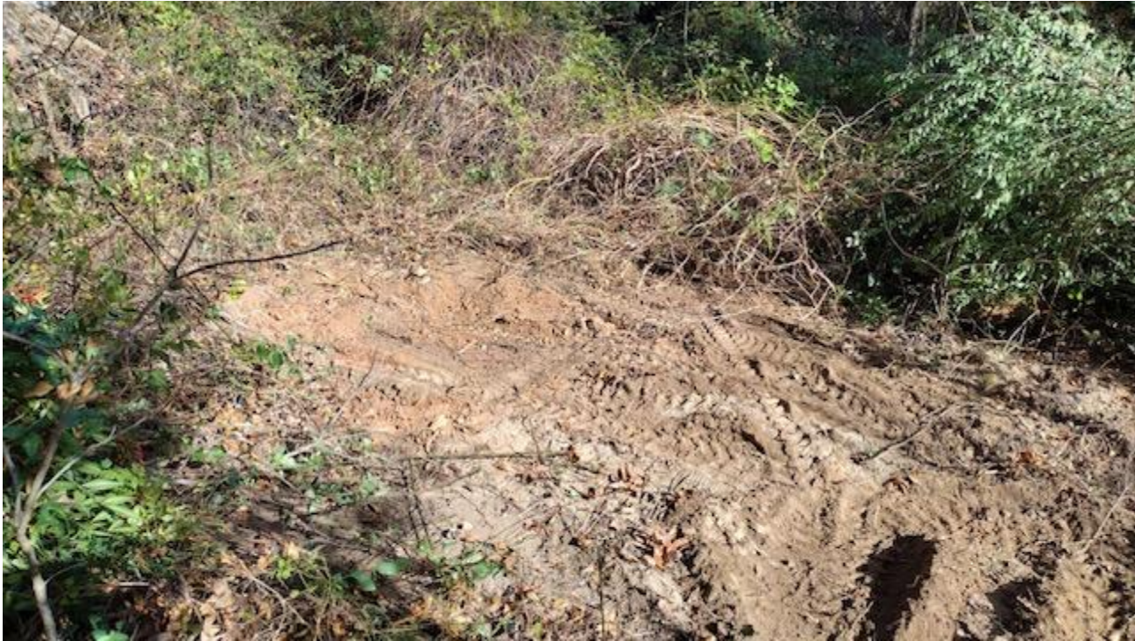
TANK COVERED BACK
