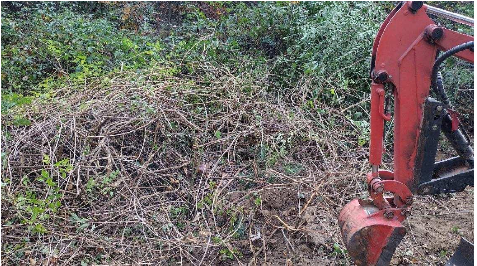
VINES COVERING TANK
