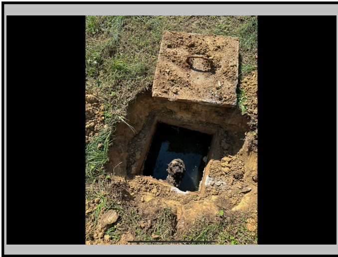
Outlet side of tank
