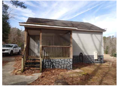
Back side of roof.
