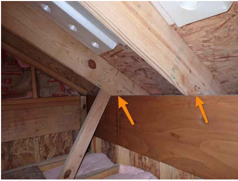
Rafter ties missing on rafters at back side of attic.
