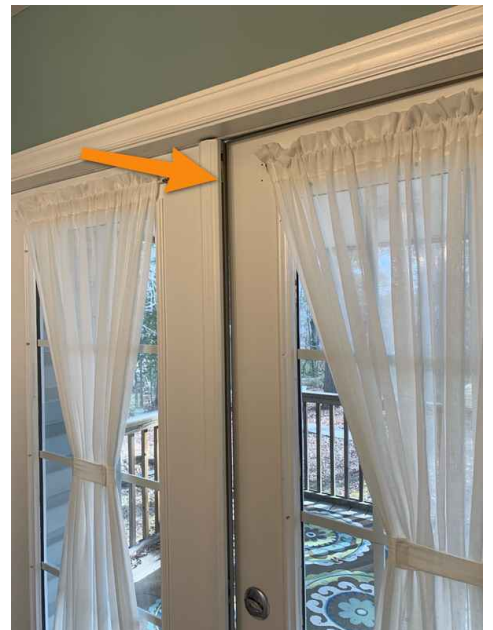
Back entry door.
