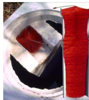
7" Filter in a 5" square concrete baffle
