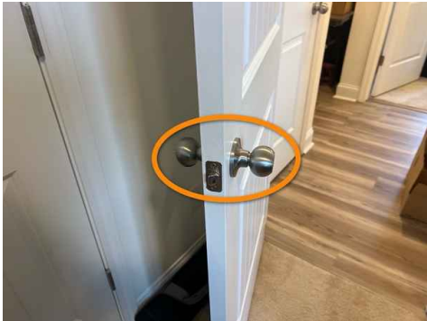
1st Floor Rear Left Bedroom
