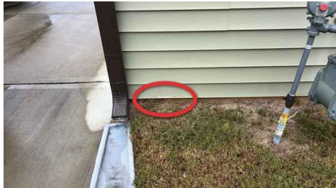
Front Right side of the house
